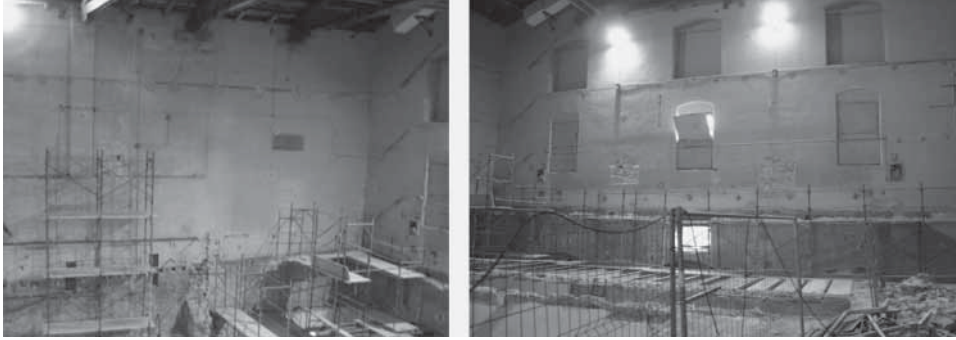
Fig. 2 - The southern wall of the fly tower (note in the lower part free of plasterwork the discontinuity between the 18 th century and 17 th century walls); the western wall of the fly tower (note the openings in the wall, besides the three big arches not in view, in the lower part under the stage).
