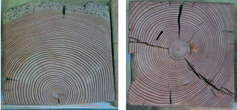
Fig. 4 - Wooden slice ZAN 1 and ZAN 5 of timber truss. The wood specie is Larch, which is traditionally considered durable (the insects attack is limited to the sapwood).
