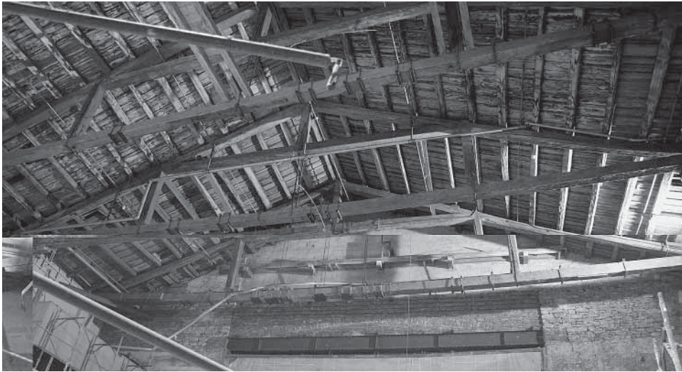
Fig. 3 - The queen-post timber truss.
